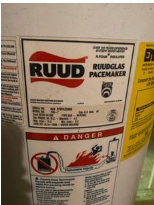
Photo Of Water Heater Dataplate
