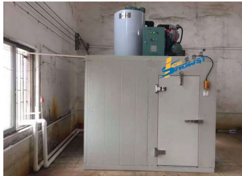
Ice Flake Machine application to Cold Storage
