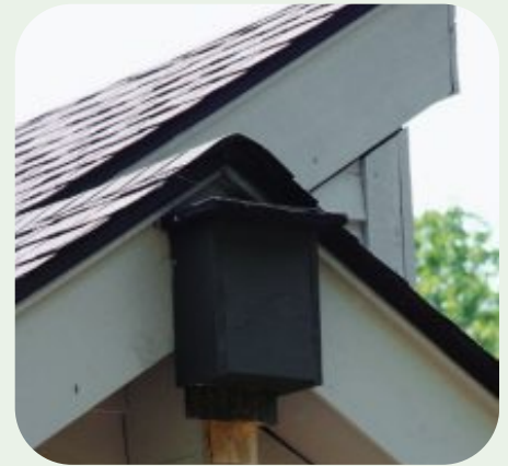
Bat box installed on roof
