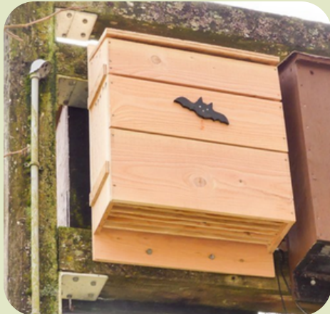
Roughened landing pad visible at the base of BCI style bat box
