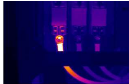
THERMAL IMAGE - HIGH TEMPERATURE FOUND IN RED PHASE
