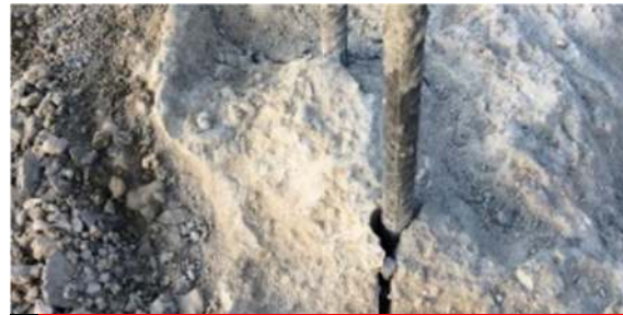
Cracks & Spallings
