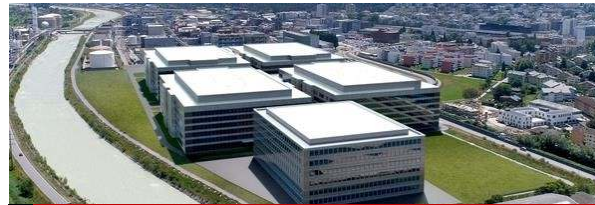
Lonza Lab – Switzerland 562 piles, Ø 1200 & 1300
