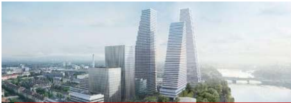
Roche Tower – Switzerland 148 piles, Ø 1200 & 1500mm
