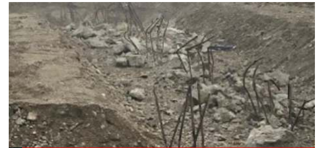
Bent / Tom Reinforcements
