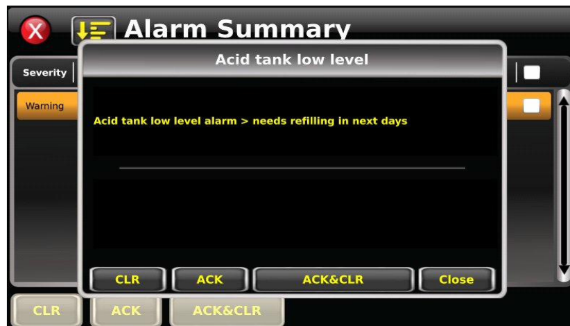
Fig. 5.2 - Alarm Info popup: detailed description and guidance for the Acid tank low level warning
