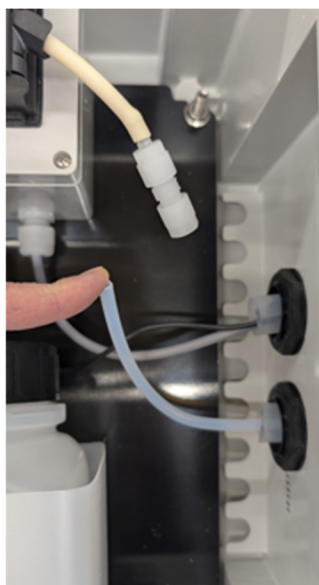
Fig. 3.5 - acid tube in acid enclosure
