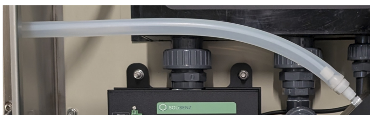
Fig. 3.6 - Acid tube fixation on non-return valve of flowcell
