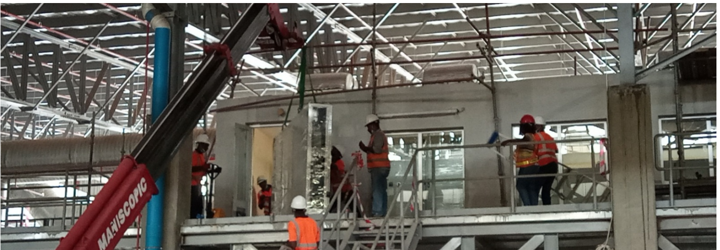
Installation of Electrical Panel
