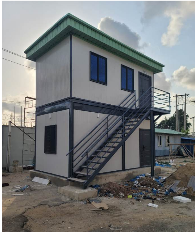
Fabrication of portacabine office
