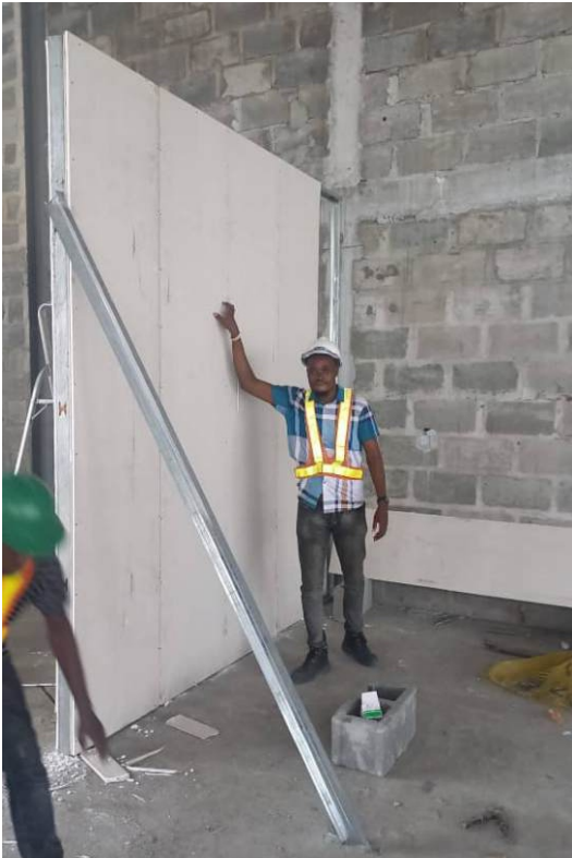
Plasters boards installation
