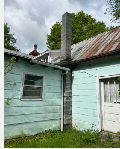
Figure 156. Corner where the 1970s addition meets the historic house, looking southwest.
