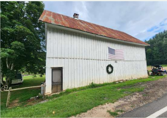
Figure 100. East elevation of store, looking northwest from NC 197 South.
