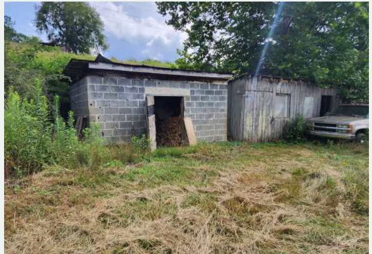
Figure 46. Concrete block and wood-framed sheds above Dove Cove Road, looking south from the pasture.
