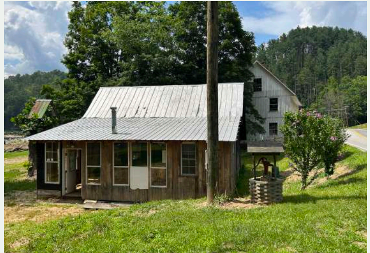
Figure 119. The store and tenant house, looking north from the yard.
