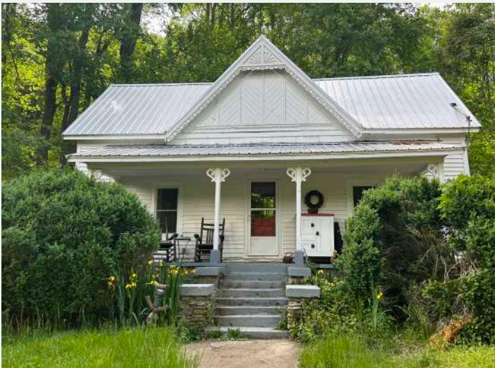
Figure 25. The Hensley-Robertson House (YC0103; 78 Riverview Road, Burnsville) reflects the Triple-A form.
