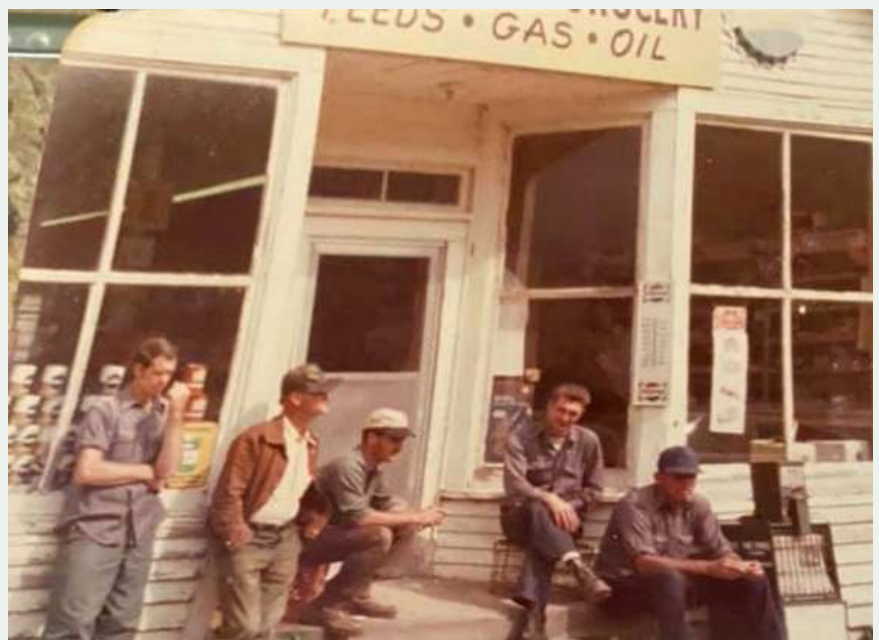
Figure 233. Men outside of the Murchison Store, 1970s. Note the change in the dimension of the reveal between the weatherboard siding above and below the windows. (Thomason, 2001)
