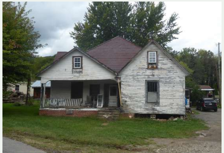
Figure 145. South façade of the Metcalfe House (YC0190).
