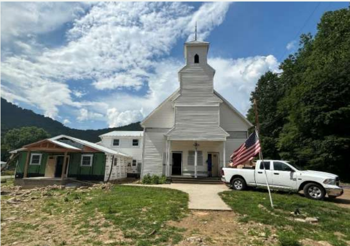
Figure 198. South façade of the church and Additions A and B to the west, looking north from the gravel parking area.
