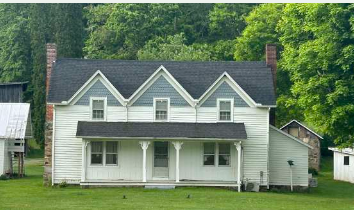
Figure 17. Horton Laughrun Farm (YC0053; 34 Gilders Creek Road, Burnsville) features tobacco and cattle barns, an apple house, sheds, root cellar and other agricultural buildings.
