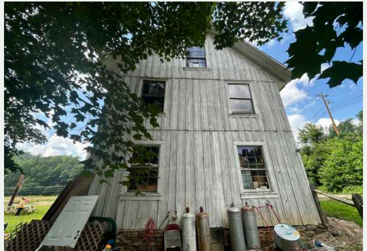
Figure 99. South elevation of the store, looking north from the yard.
