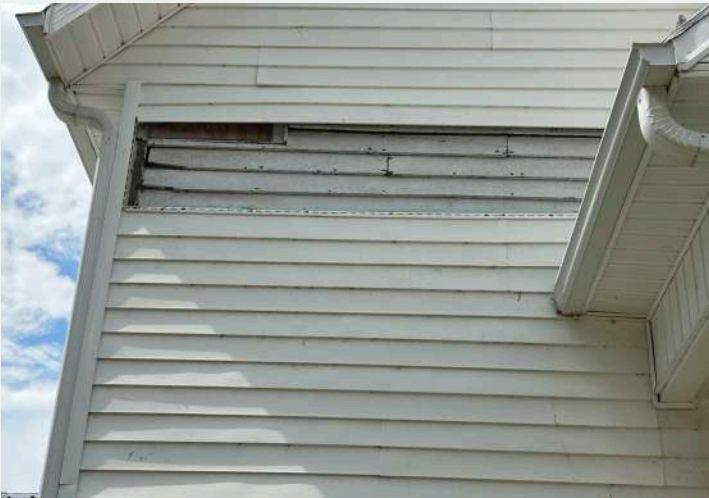
Figure 197. Historic wood siding hides beneath contemporary vinyl siding on the south facade.
