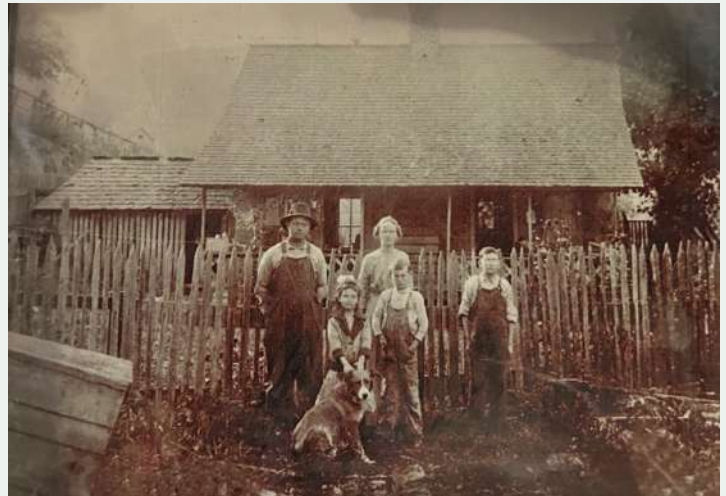
Figure 122. 1920s photograph of Bart and Sally Penland family in front of the tenant house. Note the staircase leading up to the second floor between the two front doors and the steep embankment of the railroad to the left. (D. Hensley, 2025)
