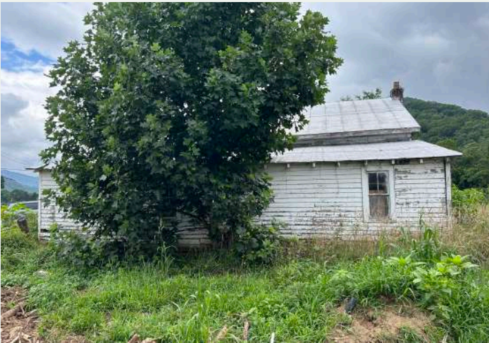
Figure 230. Northeast elevation of the store, looking southwest from the field adjacent to the building.
