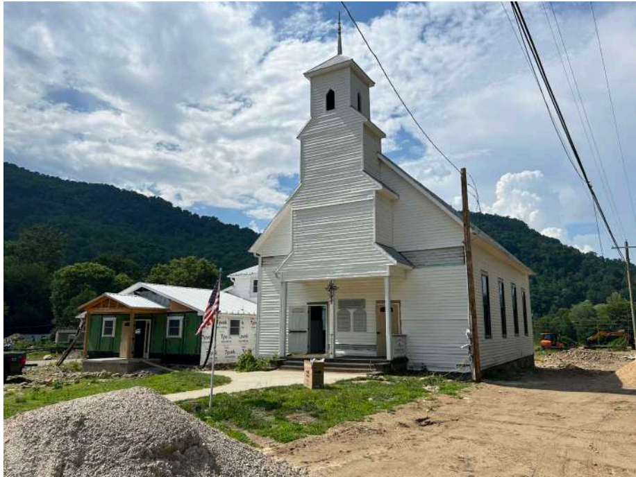
Figure 194. Oblique view of the south and east façades of the Laurel Branch Baptist Church, looking northwest from the intersection of Pensacola School Road and NC 197 South.
