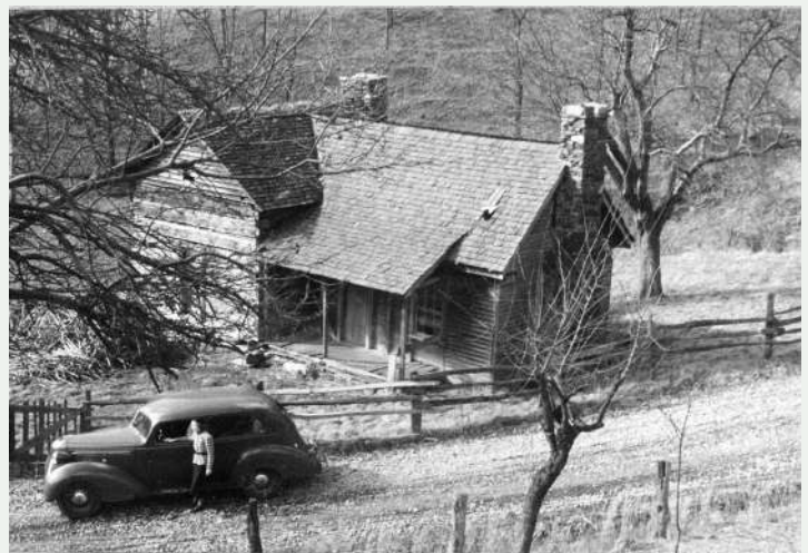
Figure 88. A circa January 1938 photograph of the Hensley Cabin, looking southwest. Note that the porch is not enclosed and the ell has narrow weatherboard siding. Split rail and post and wire fences line both sides of the road. (Sharpe, 1938)
