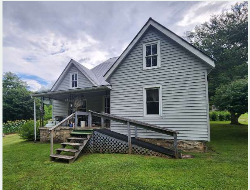
Figure 135. West façade, looking northeast from the front yard.
