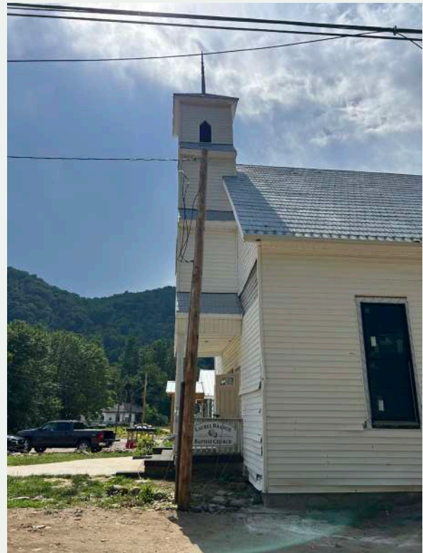
Figure 224. July 2023 photograph of the same elevation, facing west from NC 197 South.
