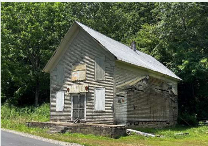
Figure 126. Oblique view of the south and east facades of the A.J. Edwards General Store.
