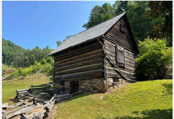
Figure 73. Granary with root cellar, c. 1812.
