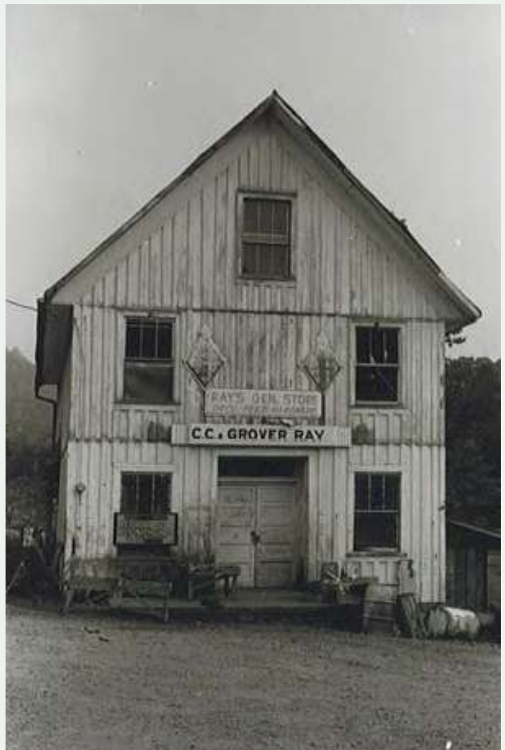
Figure 125. North facade, 1983. (Presnell, 1983(d))
