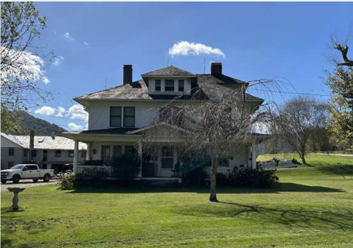
Figure 258. Northeast façade of the Joseph Wells House (BN0747).
