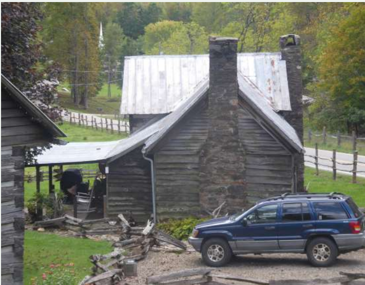
Figure 64. North elevation of the cabin, looking south from Bolens Creek Road. Note the enclosed porch addition to the left of the ell's gable end.
