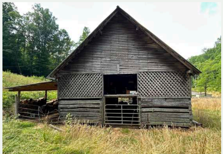
Figure 78. Transverse crib barn, looking southeast from pasture.
