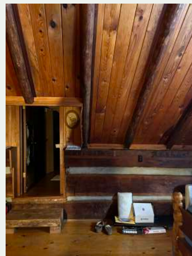
Figure 71. Looking north into the attic of the ell.
