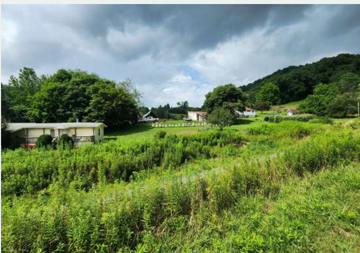
Figure 51. Overview of the site, looking north from Dove Cove Road.
