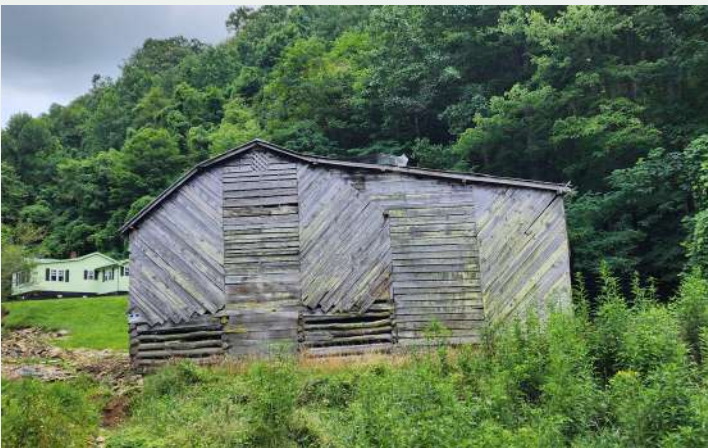
Figure 16. This barn on Hog Branch Road in Yancey County shows the evolution of barn design. The building rests on a log crib foundation with a post-1915 gambrel roof wood structure above. To the right side is a tobacco barn addition with a shallow roof slope that ties directly into the gambrel barn.
