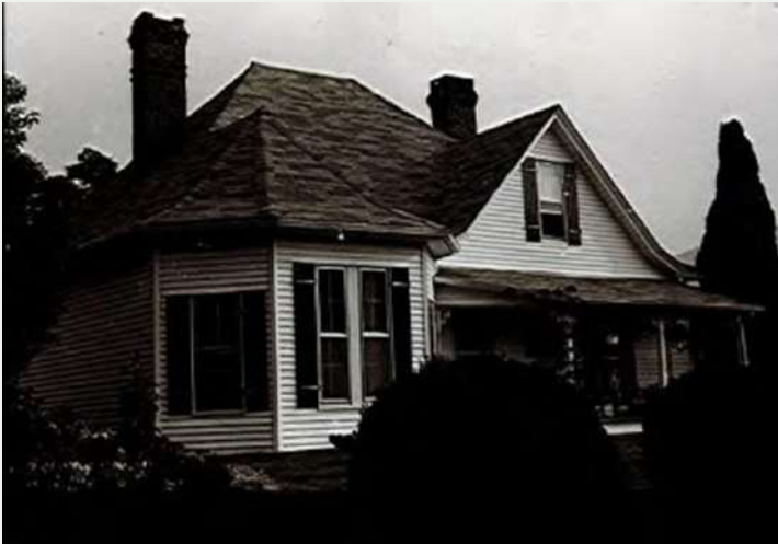
Figure 55. Oblique of the north facade and east elevation, 1983. (Presnell, 1983(a))
