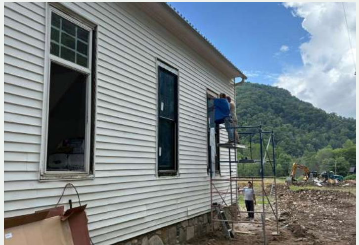
Figure 219. Church volunteers installing new windows. (Laurel Branch Baptist Church, 2025(d))
