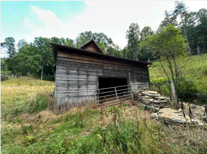
Figure 79. Tobacco barn addition, looking northeast from pasture.
