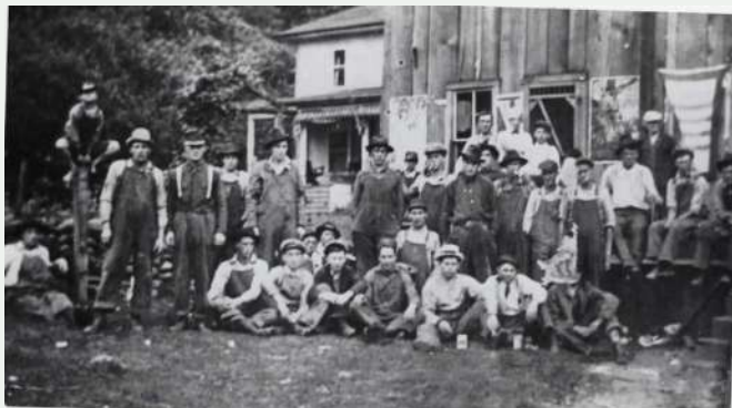
Figure 13. The Commissary stood just to the north of the Froelich House, seen in the background. (Images of Yancey, 1993)
