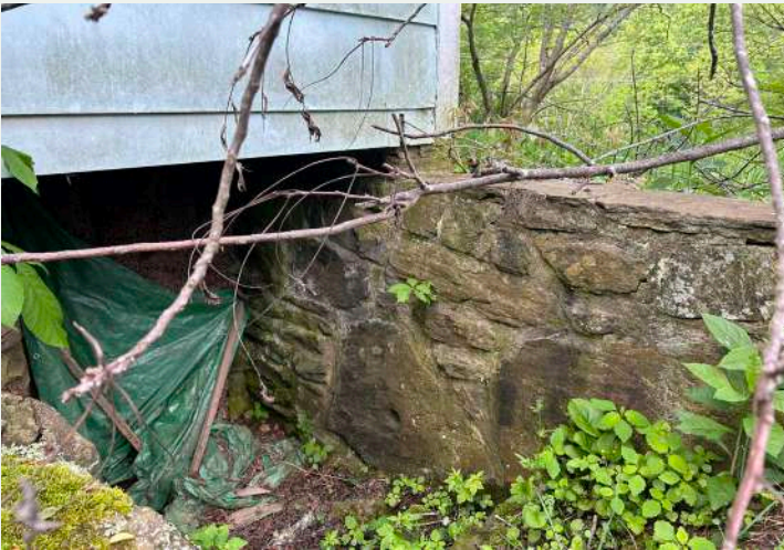
Figure 157. Cellar entrance beneath the northwest corner of the house.
