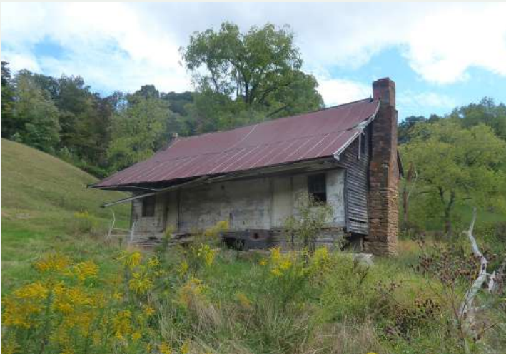
Figure 49. North façade of the tenant house, looking south from the pasture.
