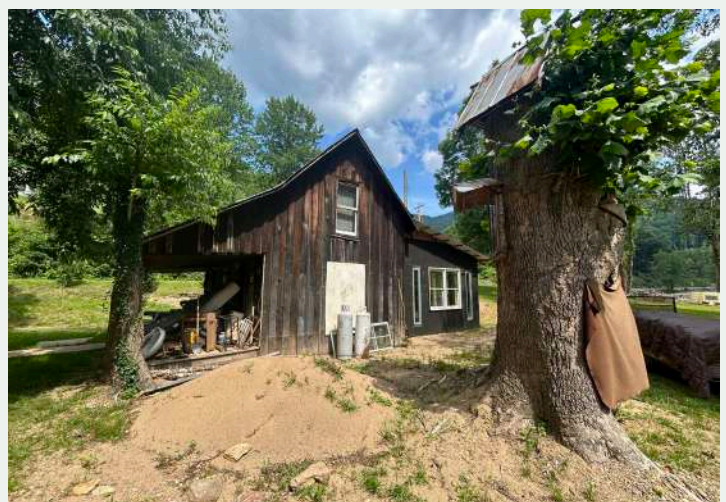
Figure 112. West elevation of the tenant house, looking southeast from the yard.
