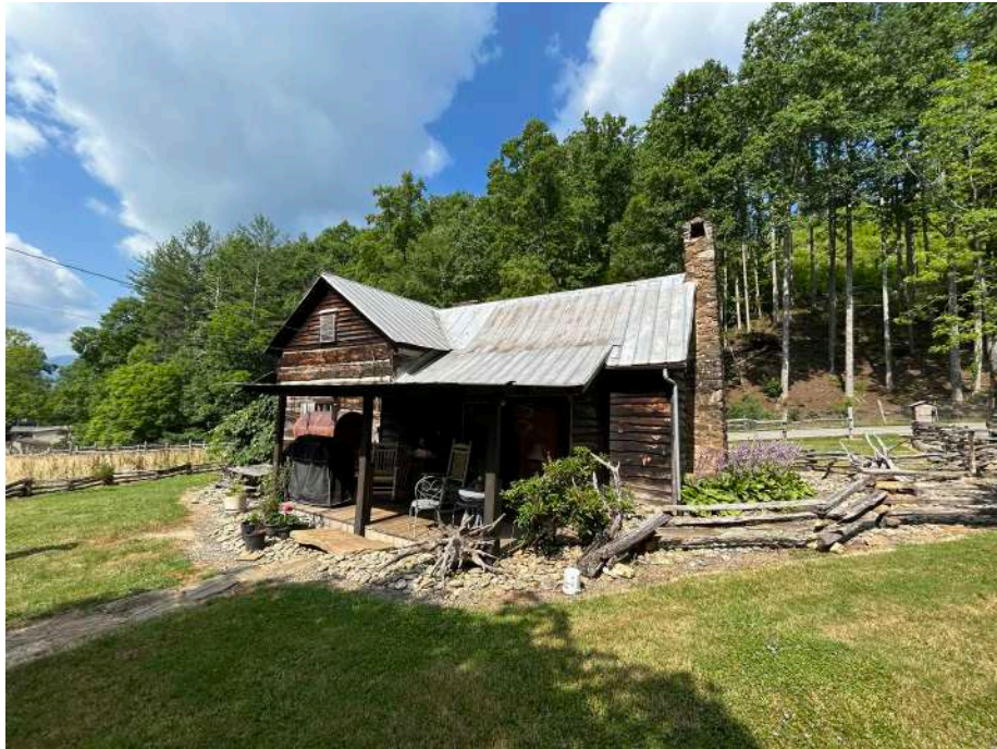
Figure 58. East elevation of the Hensley Cabin, looking southwest from the yard.
