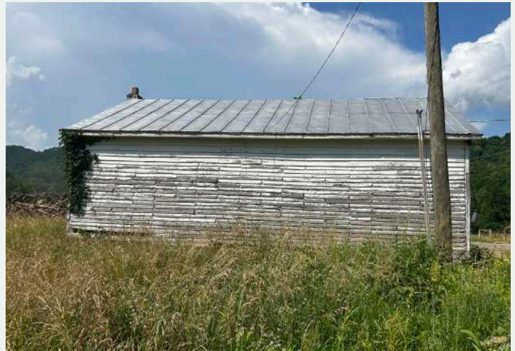
Figure 228. Southwest elevation of the store, standing on NC 197 South looking northeast.
