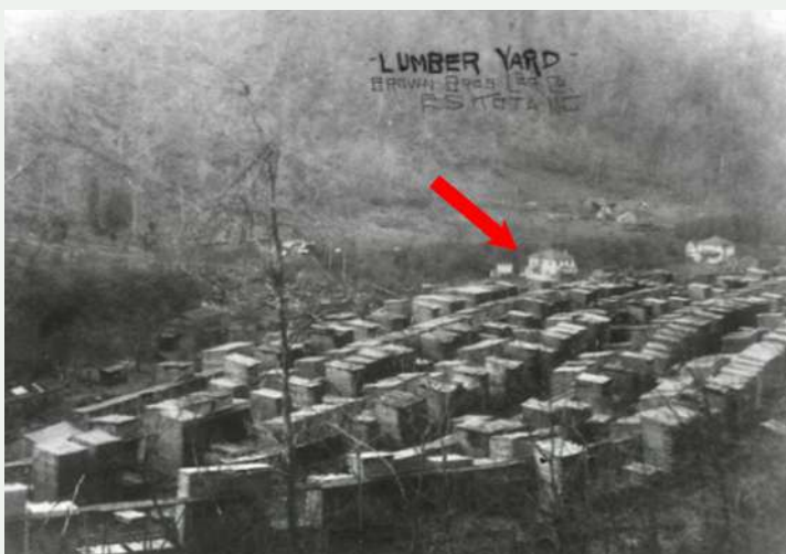
Figure 249. Brown Brothers' Lumber Company. The red arrow points to the Brown-Wilson House and shed. Note the Froelich House and commissary to the right and structures on the cleared hillside. (Childs, 2021)
