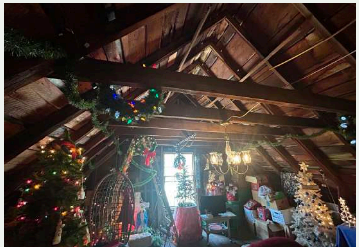
Figure 109. View of the attic, looking north.
