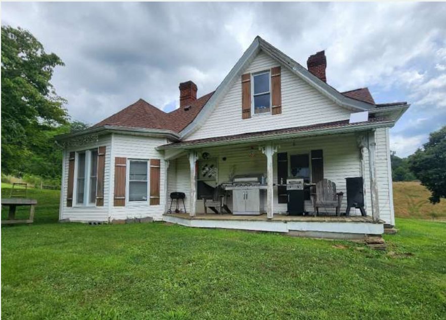
Figure 36. North facade of the house, looking south from front yard.
