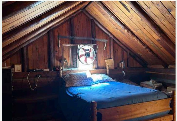
Figure 70. Inside loft, looking east.
