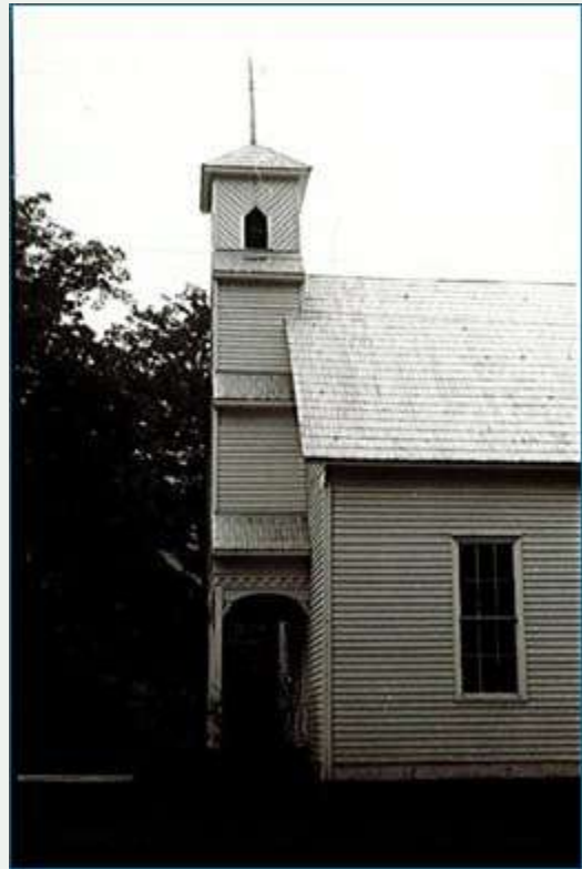
Figure 223. Circa 1983 architectural survey photograph of the west elevation. (Presnell, 1983(c))
