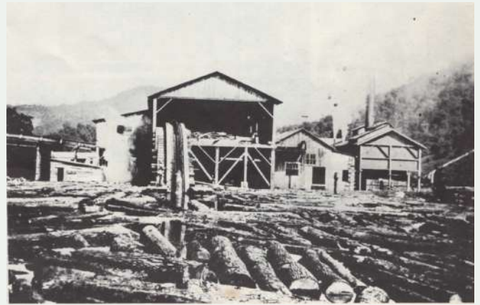
Figure 10. Carolina Spruce Band Mill at Pensacola. Logs are stored in the mill pond adjacent to the mill, waiting to be sawn. ( Common Times , 1981)
