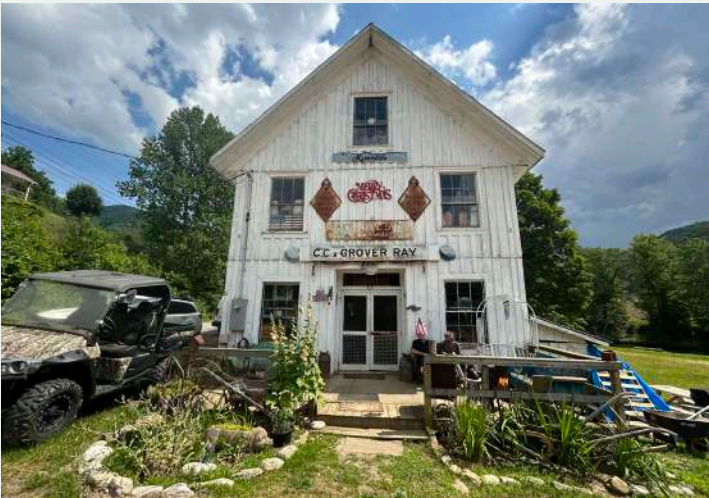
Figure 98. North facade of the store, looking south from yard.
