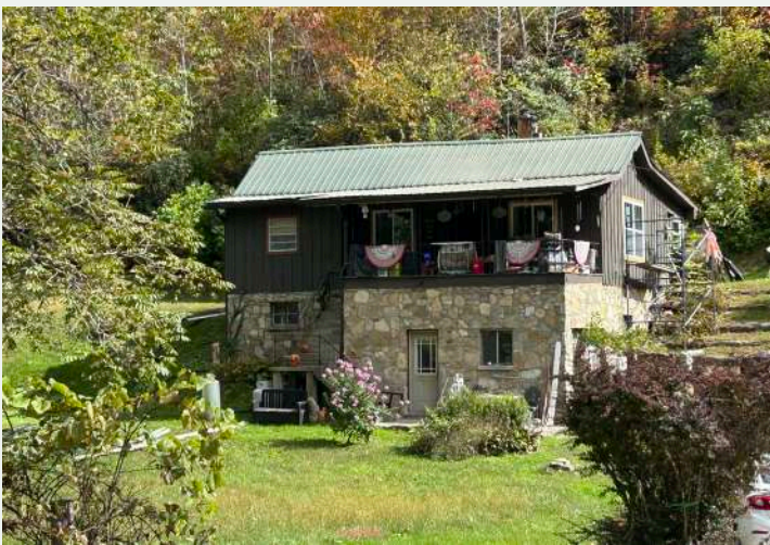
Figure 129. West façade of the Wingo House (BN6879).
