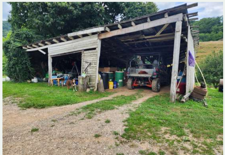
Figure 41. Three-bay garage, looking southeast from parking area.
