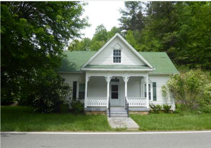
Figure 192. South façade of the Horton Maney House (YC0082).
