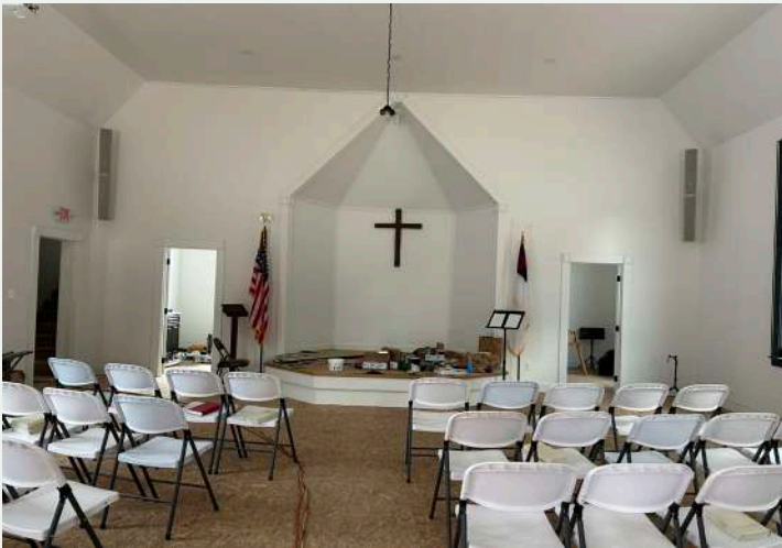
Figure 203. Interior of sanctuary, looking north. Note the particle board covering the reconstructed floor structure.
