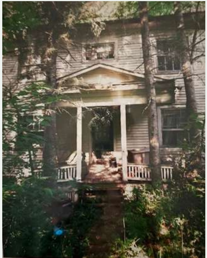
Figure 252. Front porch prior to 2001 restoration. The Boones reconstructed the porch using similar square posts but added a decorative balustrade. Note the eight-over-one windows and ten-light window above the pedimented gable. (Boone, 2025)
