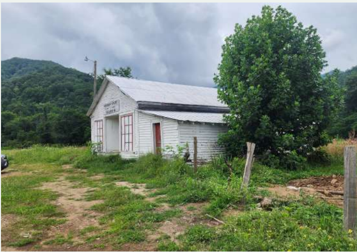
Figure 231. Oblique view of the southeast façade and northeast, looking south from the driveway.
