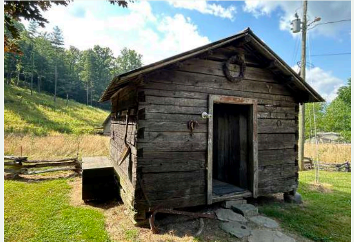
Figure 76. Smokehouse, looking south from the yard.
