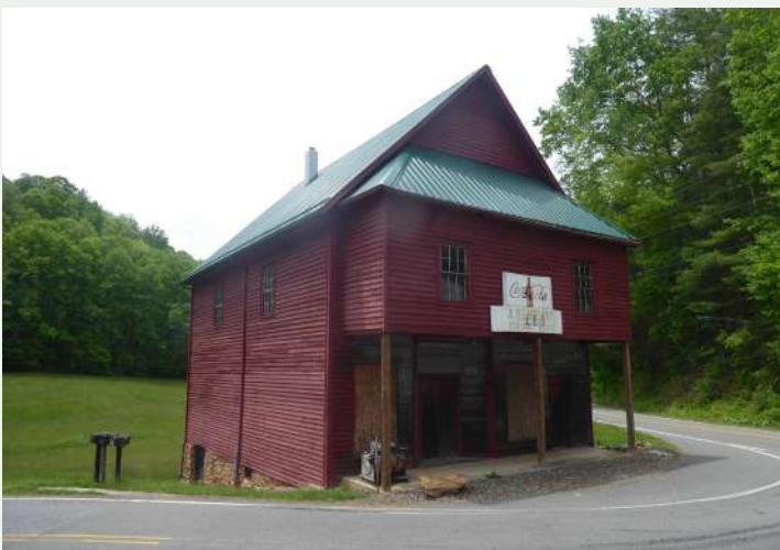
Figure 127. Oblique view of the east façade and south elevation of the A.O. England General Store (YC0048).
