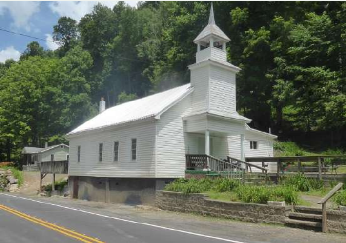
Figure 221. Oblique view of Miller's Chapel's (YC0262) south and west facades.
