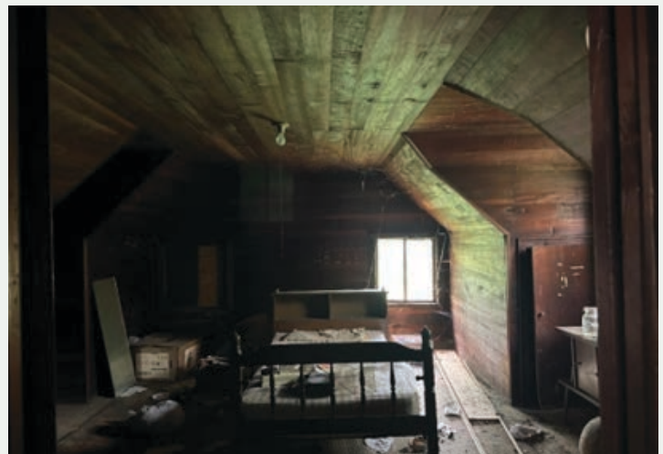
Figure 161. Bedroom, second floor, looking south from central hall.
