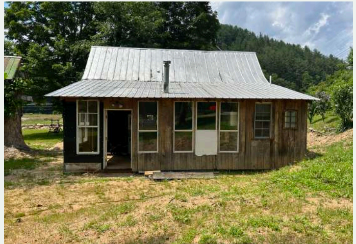
Figure 114. South elevation of the tenant house, looking north from the yard.
