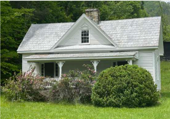
Figure 191. Southeast façade of the Henry Holcome House (YC0083).
