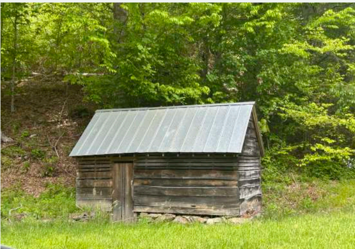
Figure 193. Shed to the southwest of the Henry Holcome House (YC0083).
