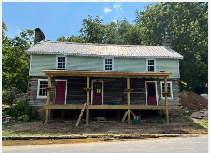
Figure 23. The Laus Peterson House (YC0177; 299 Toe River Road, Green Mountain) is an example of a nineteenth-century log cabin with an early twentieth century second-story addition, creating an I-house form.
