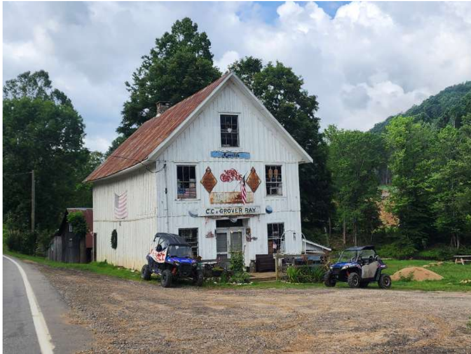
Figure 94. Oblique view of the north and east facades of the C.C. and Grover Ray Store, looking southwest from NC 197 South. Note the tenant house directly to the south.
