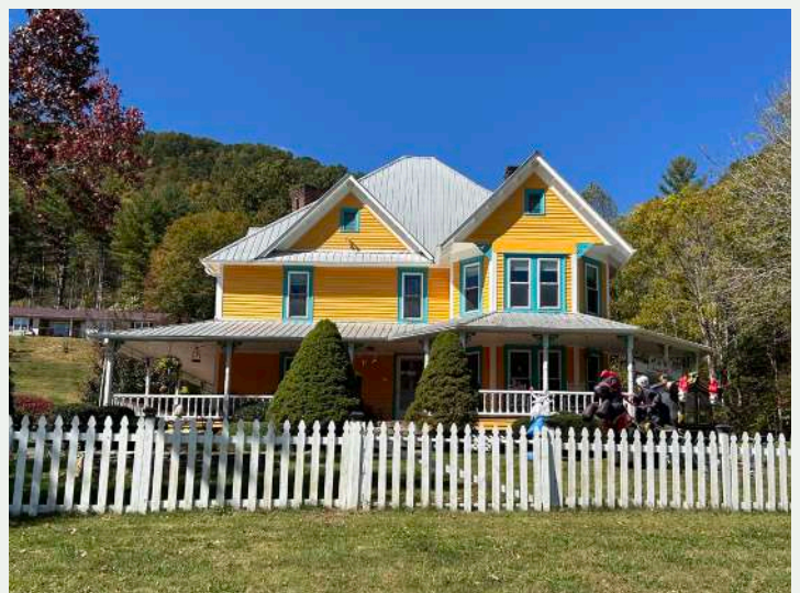
Figure 147. Southeast façade of the Dr. Peterson House (YC0091).
