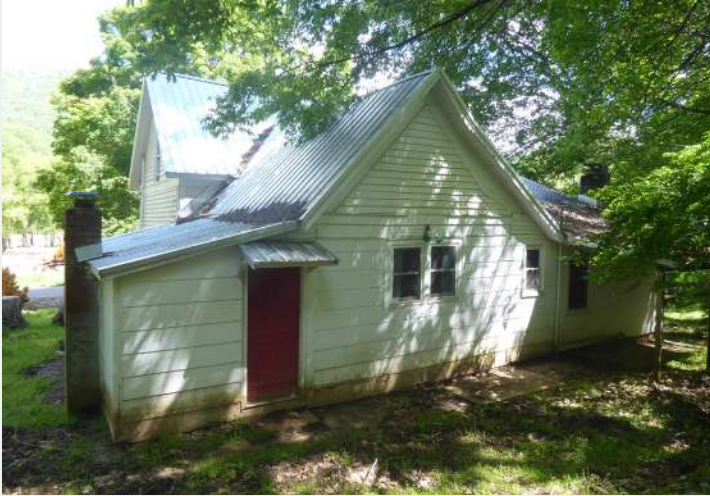
Figure 178. West elevation of the house, looking southwest from hillside. The gable of the rear ell is flanked additions A and B. Note the adjustment to the gable roof pitch on the right (south) slope of the ell and narrow weatherboard siding above Addition B's window (right).
