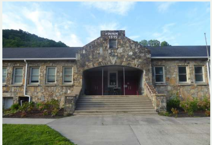
Figure 31. The Bald Creek School (YC0006; 100 Bald Creek School Road, Burnsville) reflects the WPA-era rustic revival style. Built as a high school in 1938, the building is now used as an elementary school.
