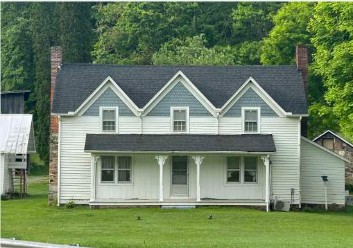
Figure 172. North facade of the Horton-McLaughrun House (YC0053).
