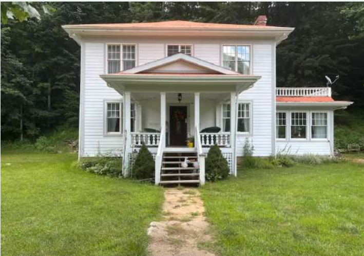
Figure 239. West facade, looking east from the front walkway.
