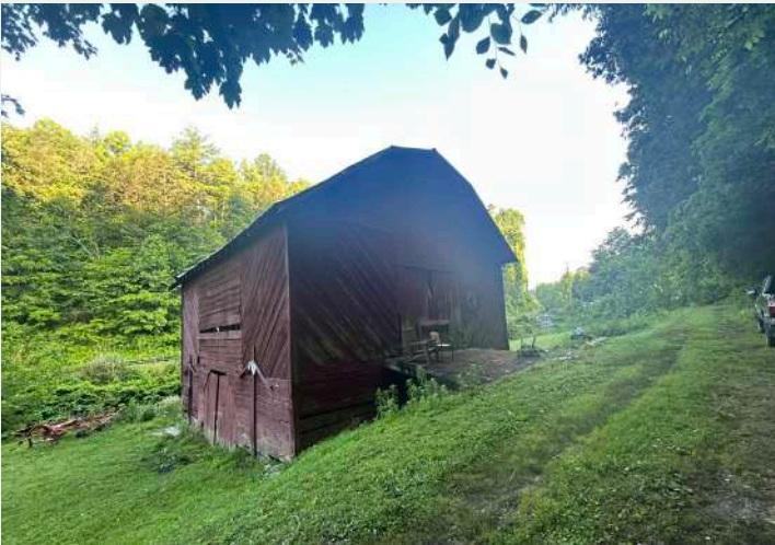
Figure 15. The barn at Hawkins Farm (MD0021; 12 Charles Blankenship Road, Marshall) is an example of a bank barn.
