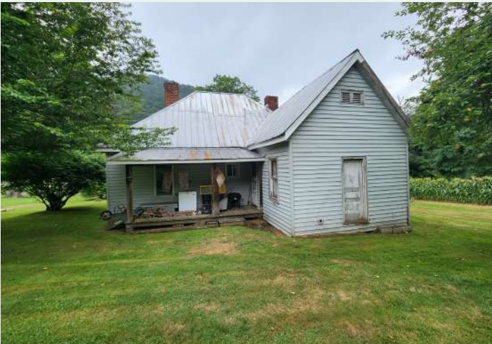
Figure 137. East elevation of the house, looking northwest from backyard.
