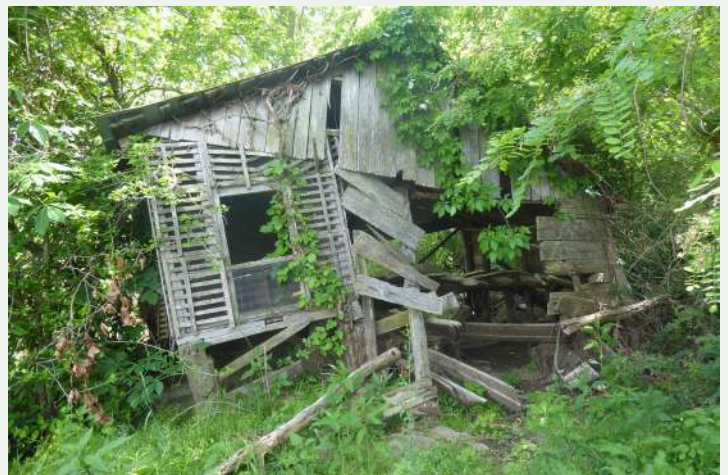
Figure 184. North elevation of the corncrib-shed structure, looking southwest from the pasture.
