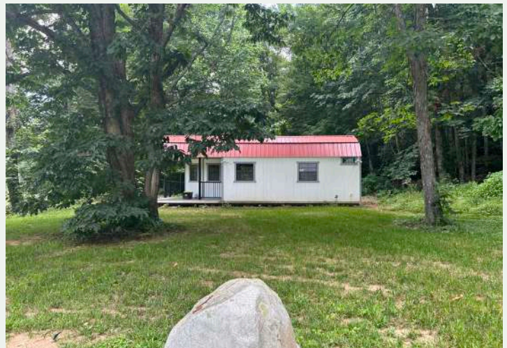
Figure 244. Tiny house, looking north from the yard.
