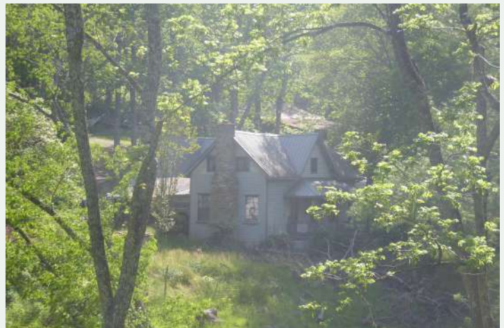
Figure 189. Oblique view of the east façade and south elevation of the Barrett House (BN2484).
