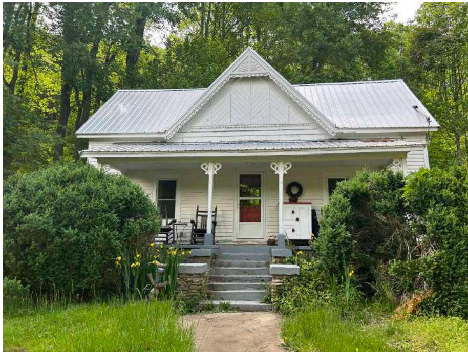
Figure 174. East facade of the Hensley-Robertson House, looking west from the front yard.
