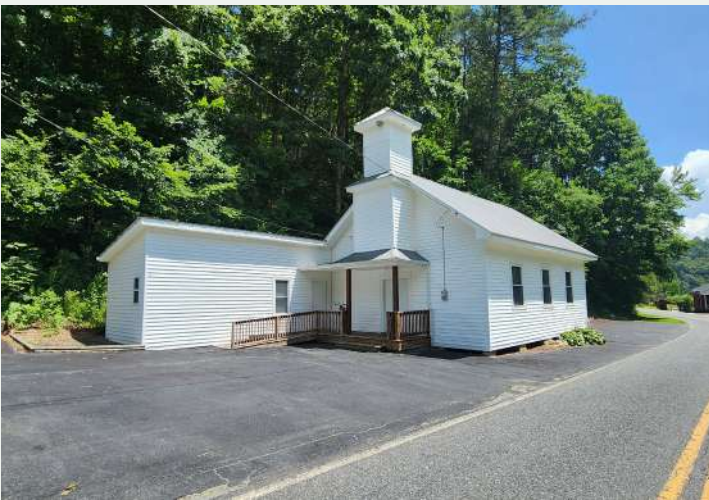
Figure 222. North façade of Brummetts Creek Baptist Church.
