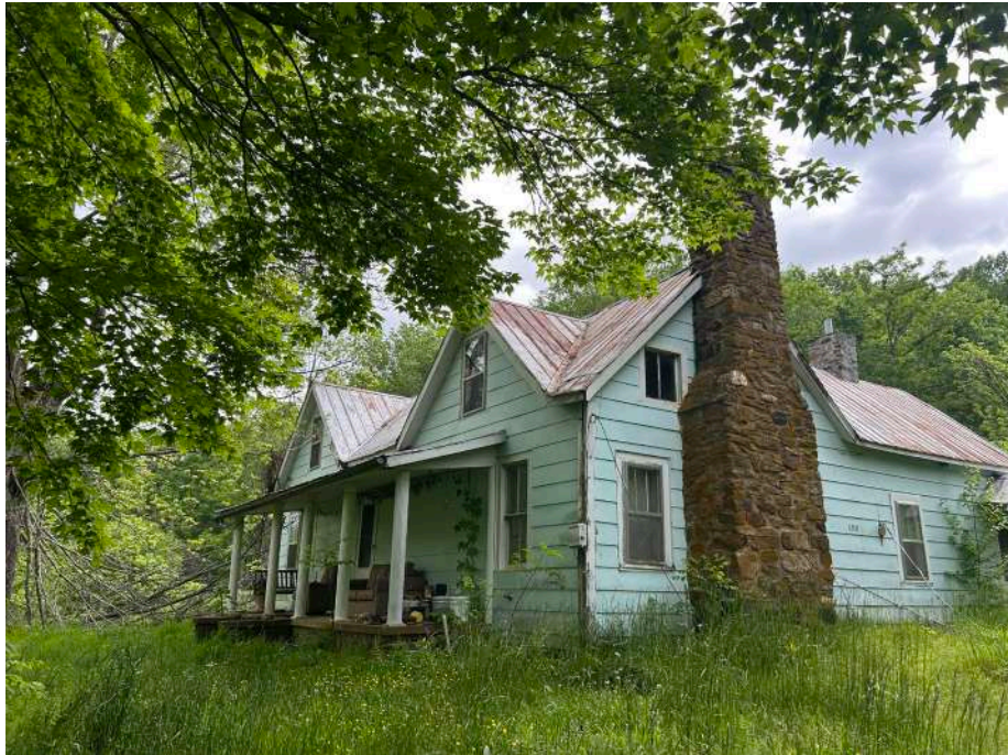
Figure 148. West and south elevations of the Joe McPeters House, looking northeast from the front yard.
