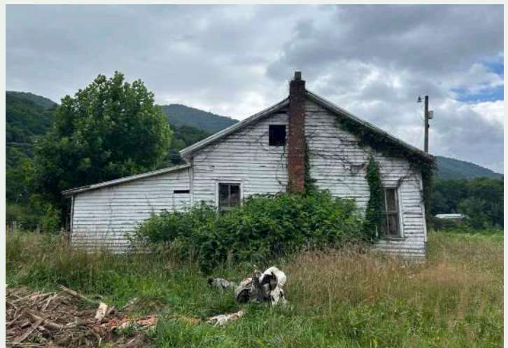
Figure 229. Northwest elevation of the store from the field behind the building, looking southeast.
