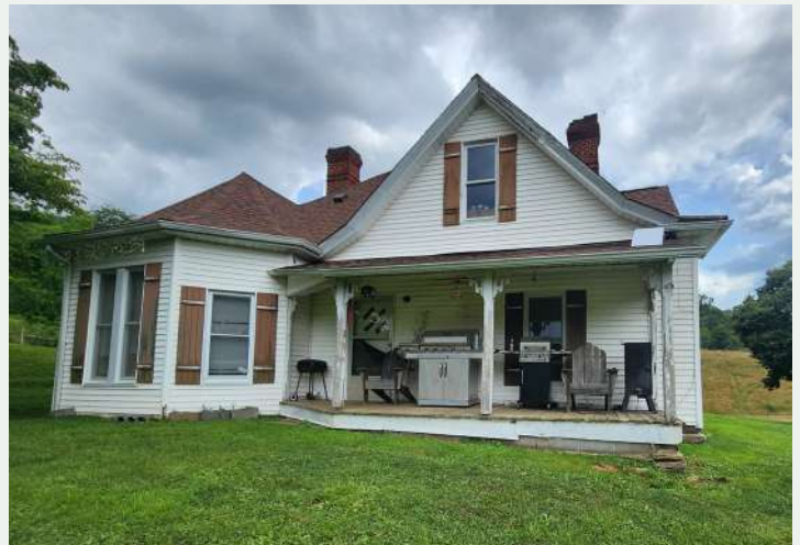
Figure 146. North façade of the David Dellinger House (YC0028).
