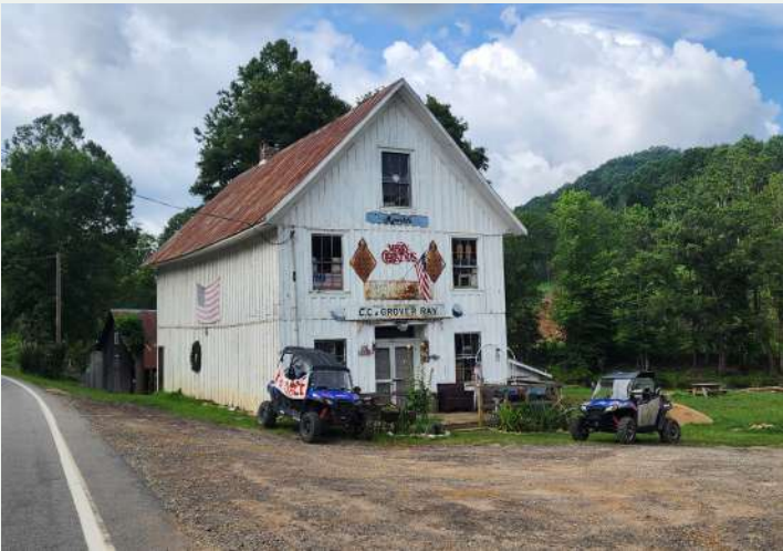
Figure 43. East facade of the barn, looking northwest from the yard.
