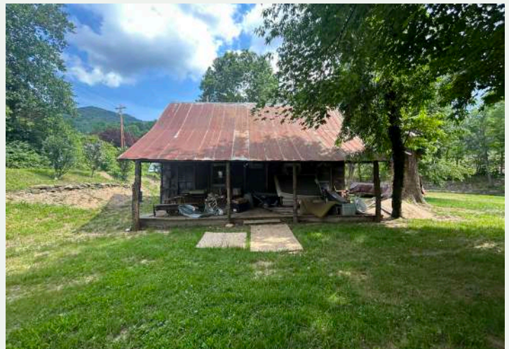
Figure 110. North facade of the tenant house, looking south from the yard.
