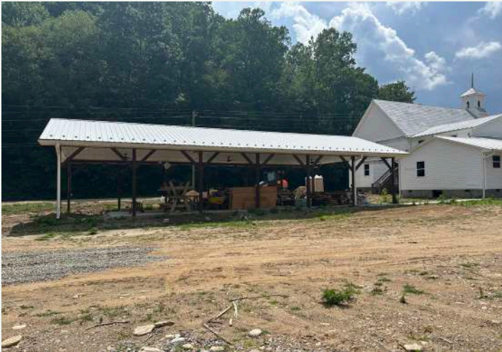
Figure 207. Pavillion, looking southeast from yard.
