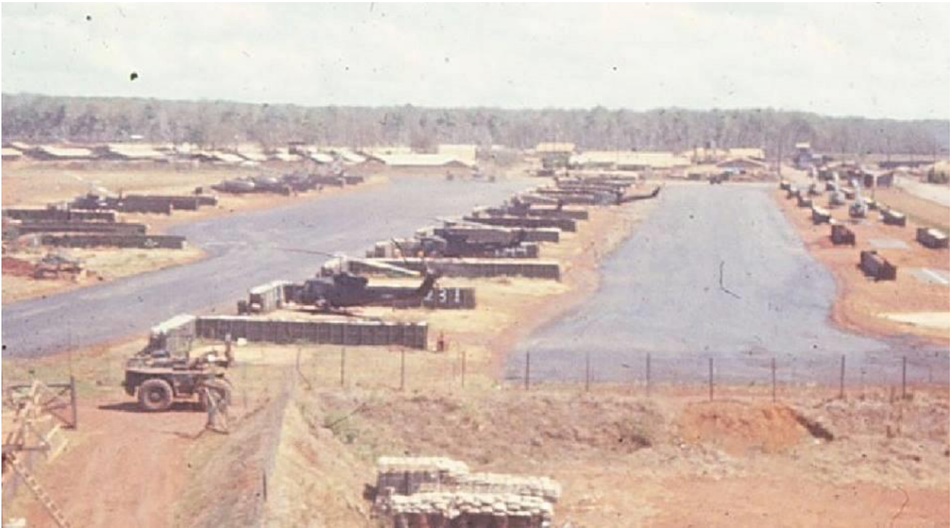
BMT City Field, on short final for landing 06 to the Corral. Center L-shaped revetments are for Falcon gunships, mostly 2 nd Platoon slicks are in open-ended revetments on either side. The runway is 50 meters or so off to the right. Circa 1969.
