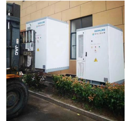
Use Forklift move to installation position
