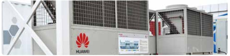
Huawei IDS1000-C series container data center solution includes independent IT, power and cooling containers for standard configuration. Meanwhile, control container and 20ft-power container are optional.
