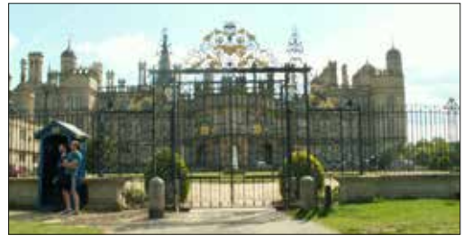
Ornate gates at front entrance to Burghley House
