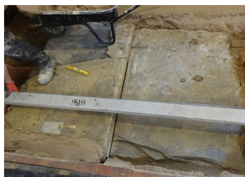
The slate slabs over vault 5. Photograph EGP
