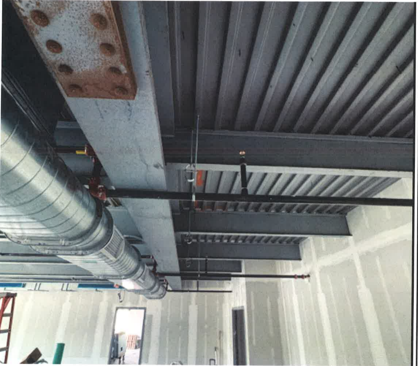
Oval Ductwork and Fire Suppression in the Gathering Hall
