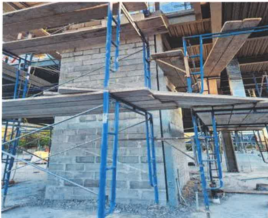
Elevator Shaft
