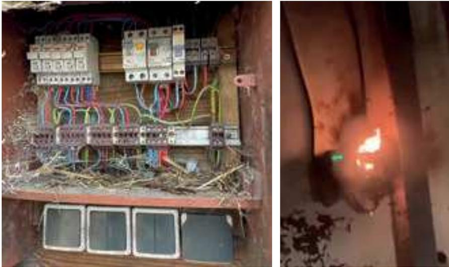
SI LES ARRIVÉES DE CÂBLES NE SONT PAS BIEN COLMATÉES, LA POUSSIÈRE ET LES DÉBRIS PÉNÈTRENT DANS LE TABLEAU ÉLECTRIQUE OÙ ILS CONSTITUENT UN RISQUE D'INCENDIE.
