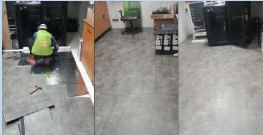
SPC FLOOR INSTALLATION - VALMET
