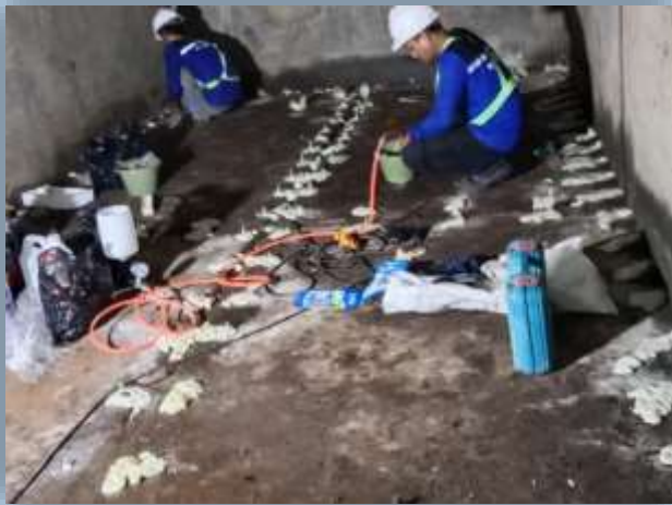
INJECTION CONCRETE – PT. SAI
