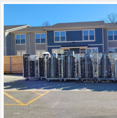
Photo 4 — Rear / Equipment Area
