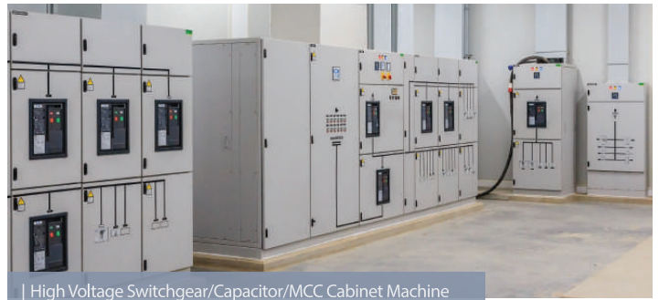
| High Voltage Switchgear/Capacitor/MCC Cabinet Machine
