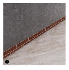
Begin the flooring installation process after the floor has been plastered. It is crucial that the finish material—whether Marble, Granite, or Porcelain—extends to the brick level.
