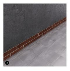
Begin the flooring installation process after the floor has been plastered. It is crucial that the finish material—whether porcelain or ceramic tiling—extends to the brick level.
