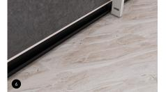
Begin this step by installing the MRG-001 Profile. First, measure and cut the profile to match the dimensions of the space using an aluminum blade miter saw.
