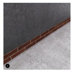
Before installing any finish materials, ensure that the last 20 cm of plastering is removed or not plastered from the beginning. Typically, you leave 10 cm from the Floor Finish Level (FFL) unplastered, resulting in a total of 20 cm from the concrete level
