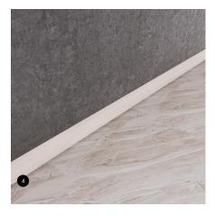
After the installation of the finish material and ensuring it is level, proceed with installing the profile using tile adhesive. To enhance adhesion, consider adding 10% of 'Addibond' to strengthen the attachment to concrete.
