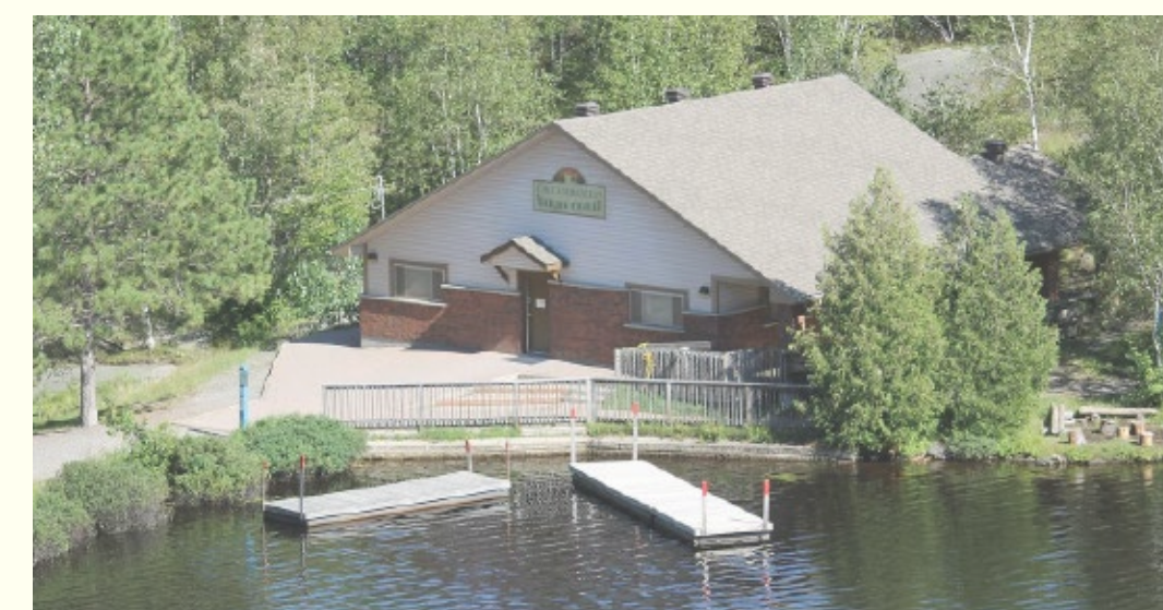
(Left) The Nature Chalet: This is the existing facility on site used as a place for learning in a natural context, used year round to host summer camps and school workshops. This design project aimed to create a larger space with new amenities. (Photo courtesy of Lake Laurentian Conservation Area, Facebook, 2020.)
