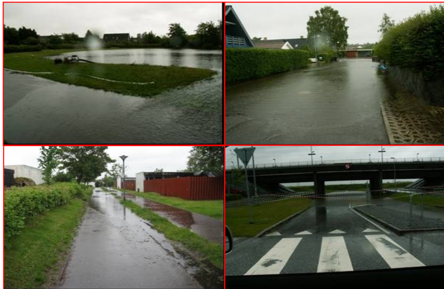
Figure 11: Aspects of the physical damages in Egedal on 13-06-2009.
