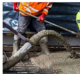
Pumped Concrete
