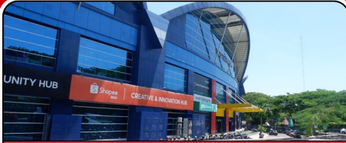
Solo Techno Park Jebres Jebres Surakarta Paving Holland K300/8cm
