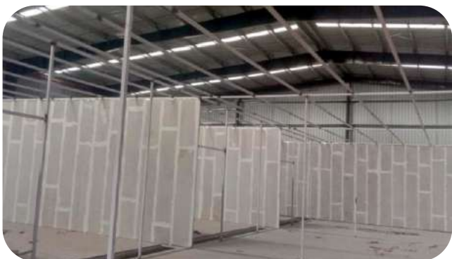
Internal Partitions / Rapid construction
