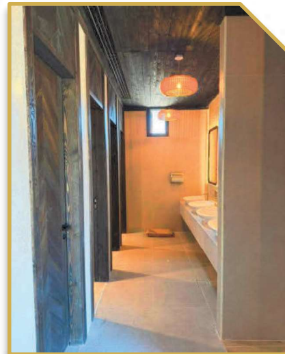
Washroom Facilities — Sink Counter Row & Woven Pendant Lighting
