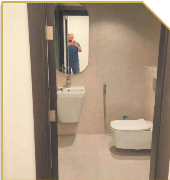
WC Cubicle — Wall-Hung Pan, Concealed Cistern & Handheld Bidet
