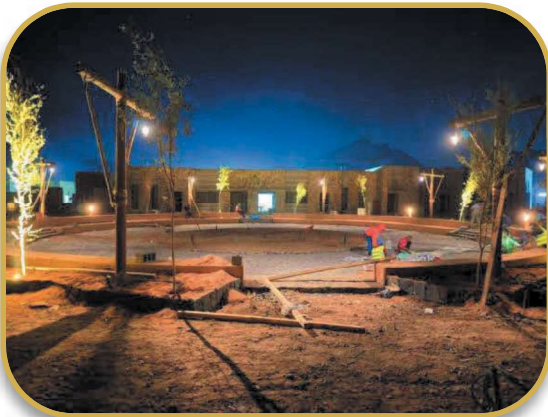
Circular Amphitheater Under Construction — Night Work & Cobblestone Paving
