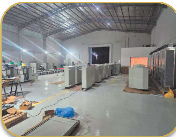
Production Floor — Electrical Panel Assembly · Rows of MCC Switchgear
