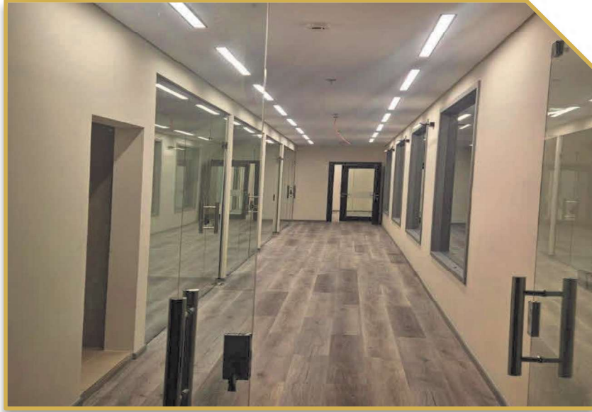
Internal Corridor — Full-Length Frameless Glass Partitions · Continuous LED Strip Lighting
