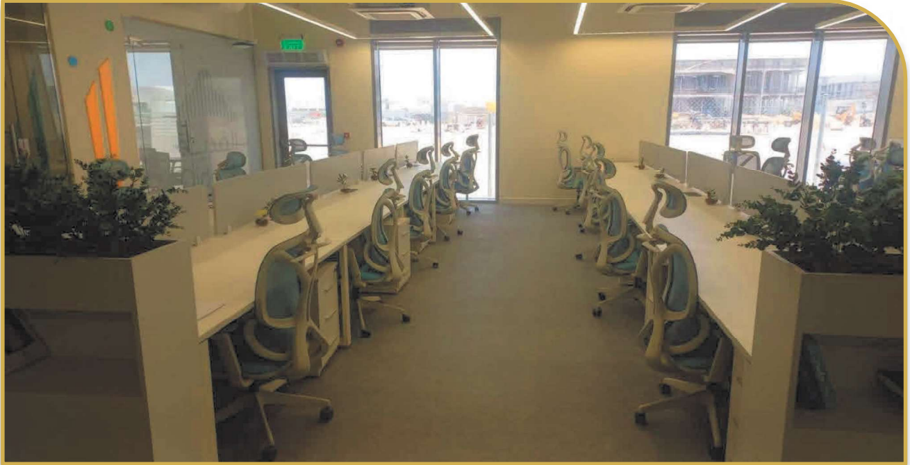
Open Workstation Floor · Electrical Distribution, HVAC & Low Current Systems
