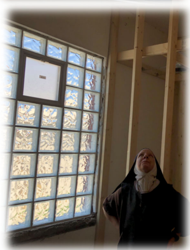
Sr. Clare looking over what will be the new shower room
