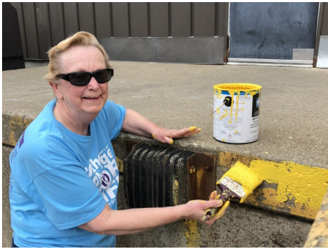
Ruth painting the concrete on the ramp of the RGM so the delivery trucks can see the boundaries!
