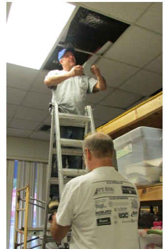
Installing new brighter lights
