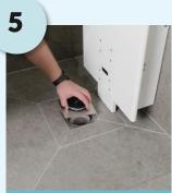
INSERT the LOOP drain cover
