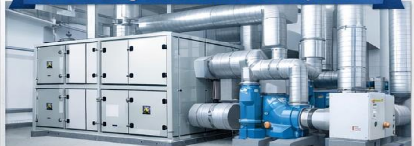
Air Handling Units & Chilled Water System
