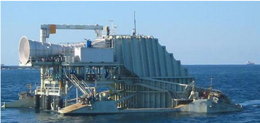
Figure 25 Oscillating water column 119
