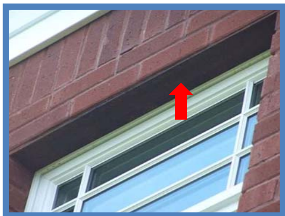
Steel Lintels found on Brick Veneer
