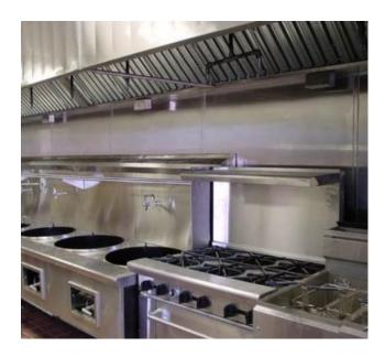
This photo shows a nice new commercial kitchen. Baffle filters and AES nozzles are in place in the hood. But....do you see any problem with this cooking line?
