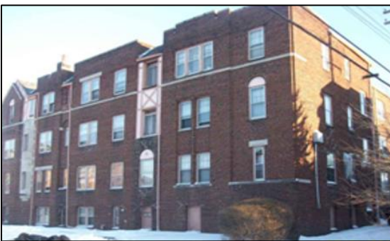
Solid brick exterior walls
