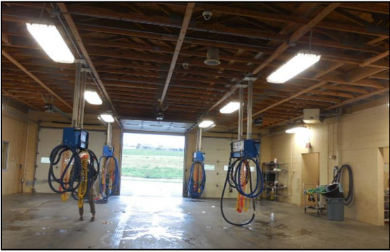
Example of ISO-2 Interior: Concrete block load-bearing walls with wood roof supports.
