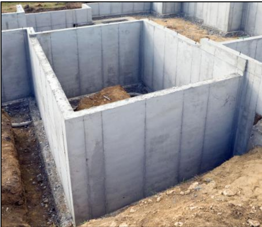
Poured concrete basement walls
