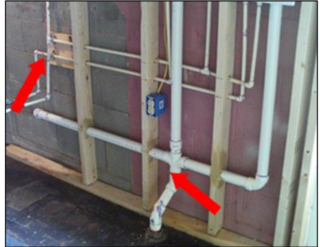
PVC supply lines and PVC waste lines
