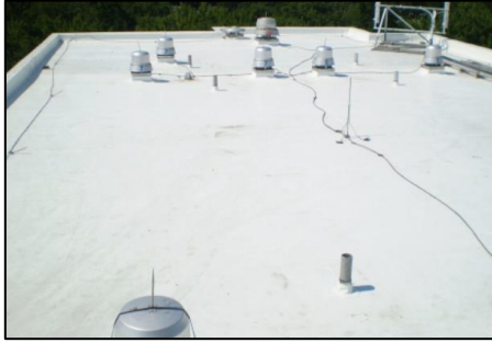
Rubber (EPDM) Roofing
