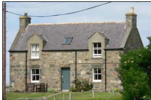
Solid stone exterior walls
