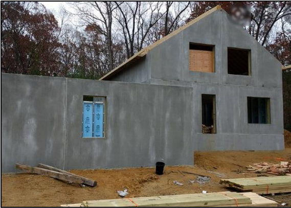
Precast concrete exterior walls with wood roof supports.
