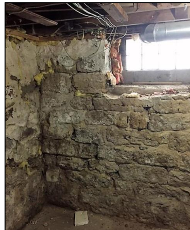
Solid stone basement foundation walls.
