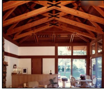
Wood/Timber Roof Trusses
