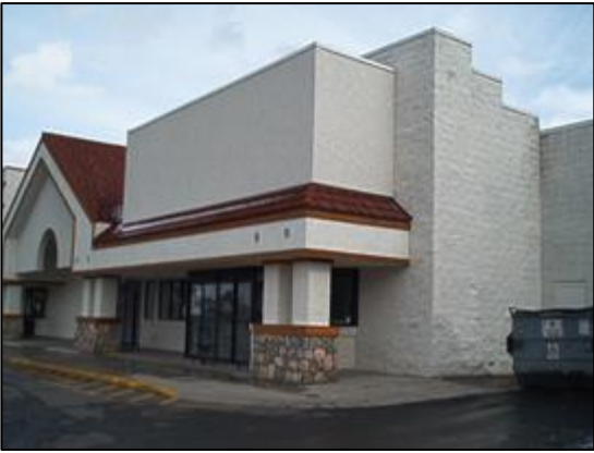
Concrete block exterior walls
