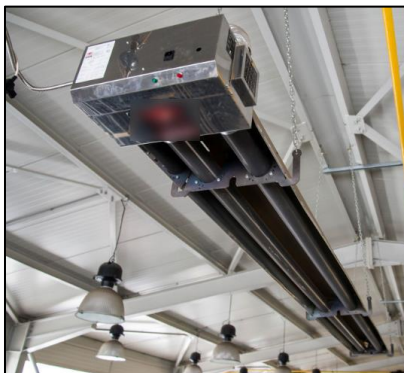
Radiant gas heater
