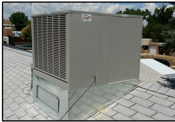
Evaporative Cooler (Swamp Cooler)
