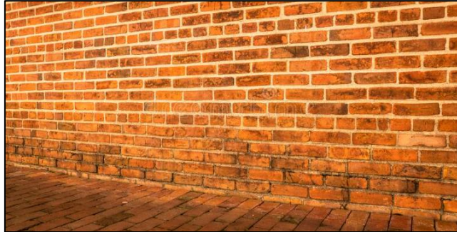
Solid Brick-No weep holes.
