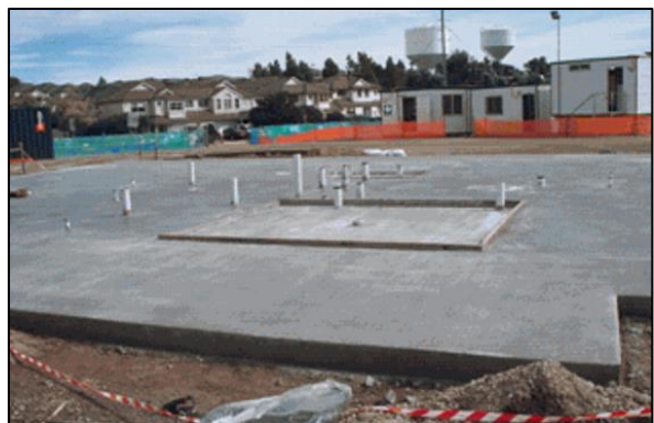
Concrete slab poured over footers
