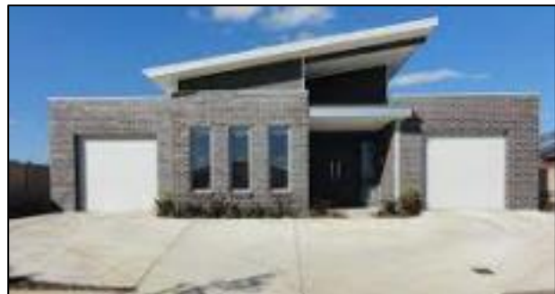
Combination Flat & Shed roof
