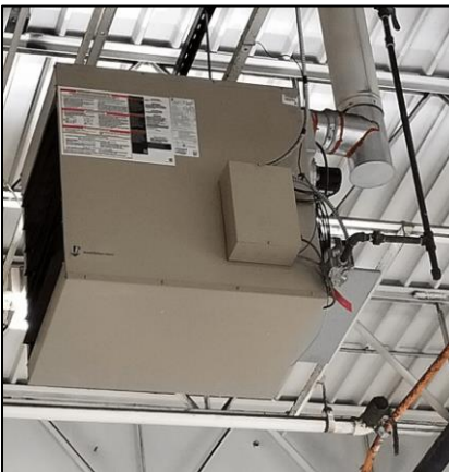
Suspended Forced Air Heater - Gas
