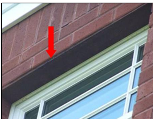
Brick Veneer: Steel lintels above the windows.
