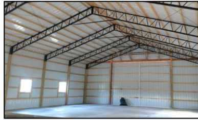
Steel Roof Trusses/Beams
