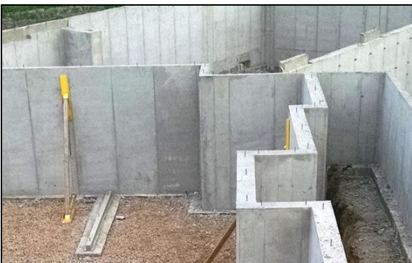
Poured concrete exterior walls.
