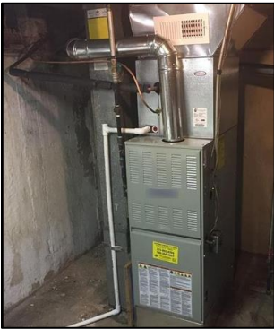
Forced Air Furnace – Gas
