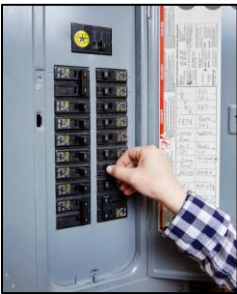
Circuit Breaker Panel Box
