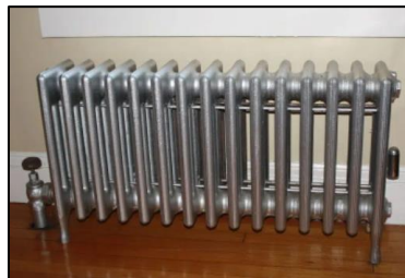
Hot Water/Low Pressure Steam
