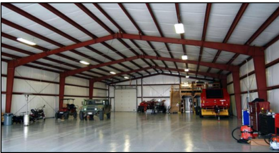
Pre-engineered metal structure
