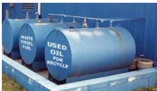
Note the secondary containment
