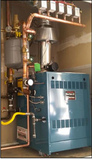
Hot Water Boiler – Gas-fired
