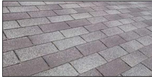
Asphalt/Composite Shingles
