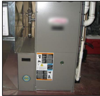
Forced Air Furnace – Electric
