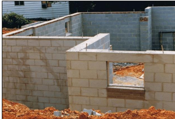
Concrete block basement walls
