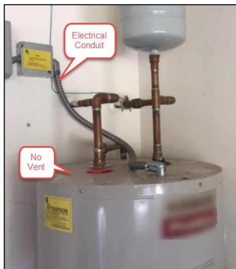
Electric Water Heater
