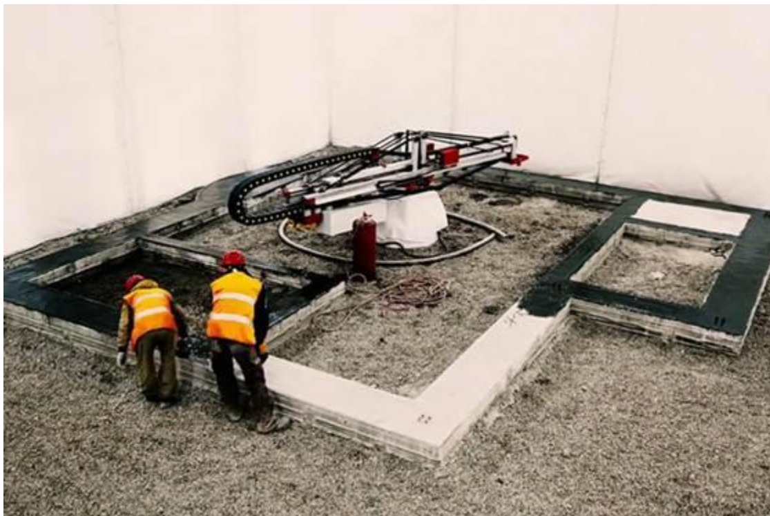
Figure: A mobile robotic 3D printer constructing the concrete walls of a small house (Apis Cor project). Such automation can erect a building's shell in hours, with minimal human labor, heralding a future of dramatically lower construction costs.
