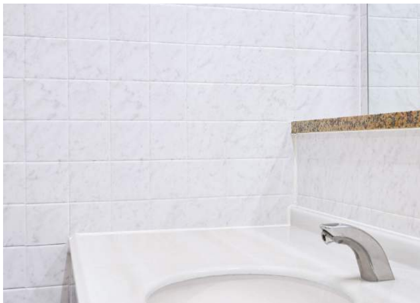
Restroom refurbishment / ST-024TIL
