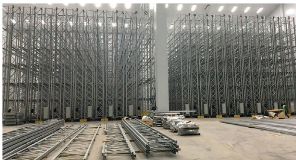
Mobile Racking during installation.
