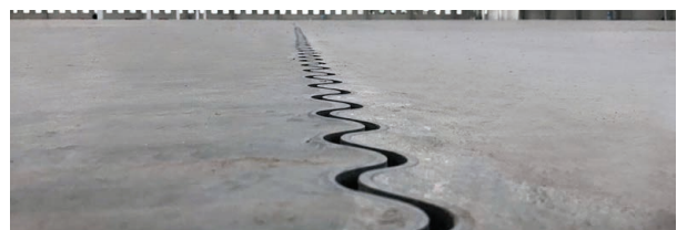
Example of a cosine joint.
