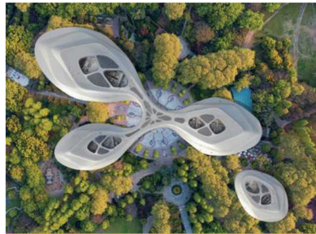
PV System Project Hainan, China | Year: 2019
