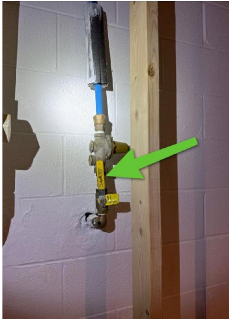
Gas/LP: Gas Shutoff Valve Information
