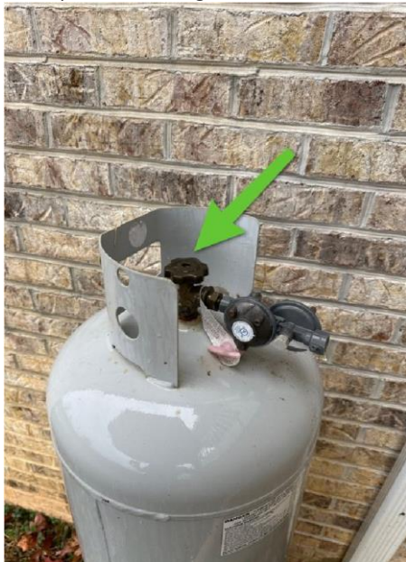
Gas/LP: Gas Shutoff Valve Information
