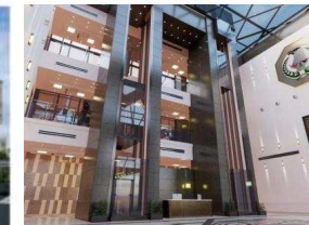
IRAQ BAGHDAD MINISTRY OF INTERIOR MAIN OF DATA CENTER
