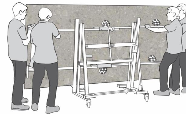
Large format Adicon SLABS always require back-buttering. Back-buttering describes the process of applying a layer of adhesive to the back of the tiles using a trowel.
