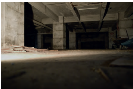
Roland Bauer Installation
