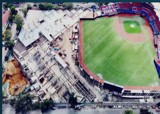
Construction of the Oaxaca Warriors Baseball Stadium, Oaxaca, Oaxaca de Juárez
