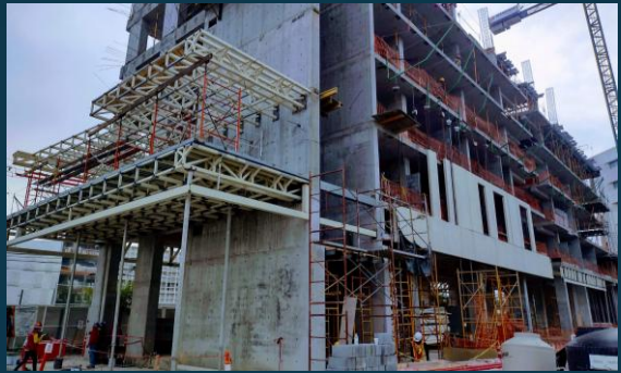
Construction of student dormitories for the Monterrey Institute of Technology, Monterrey, Nuevo León
