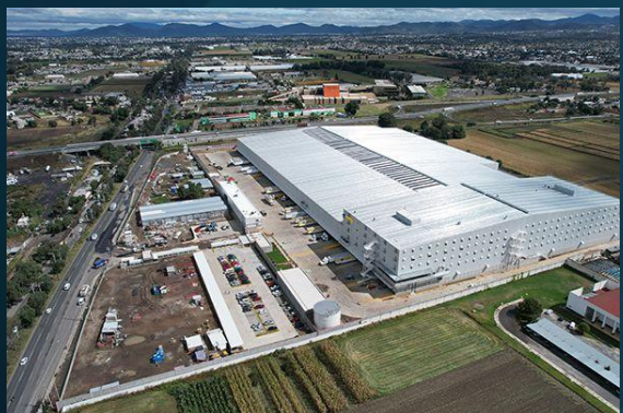
Construction of Coppel distribution center, Texcoco, State of Mexico
