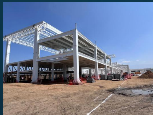
Construction of the Oaxaca International Airport, Oaxaca, Oaxaca de Juárez
