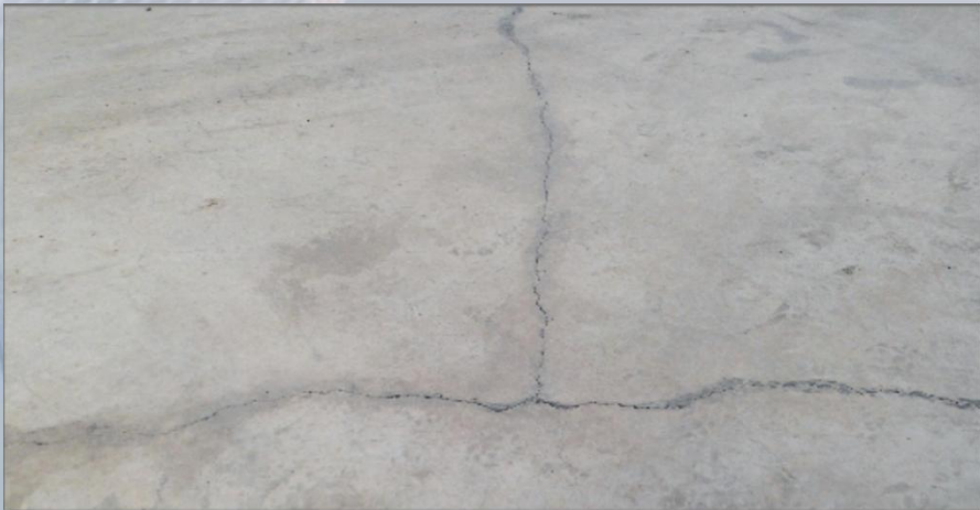
Penetration Reinforcement for Concrete Cracks
