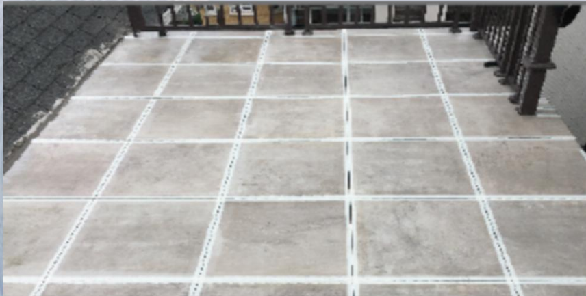
Tile Roofing Non-Invasive Waterproof Repair
