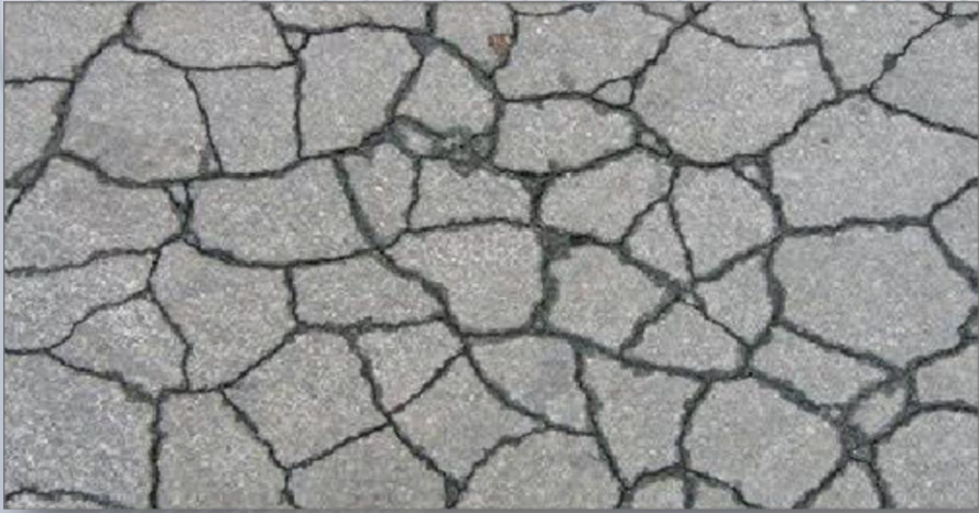
Closure of Concrete "Spider Cracks"
