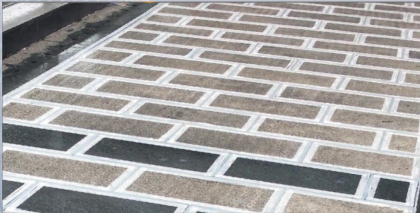
Non-Invasive Leak Repair for Terrace Joints
