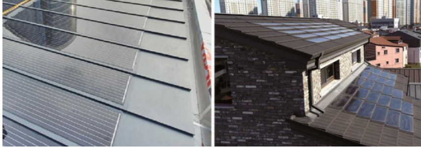
Integral Roof BIPV Construction
