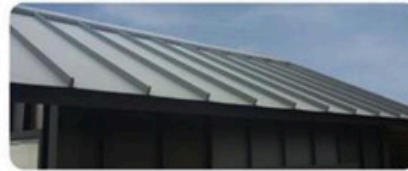
Case study of eaves finishing without installing a water catcher
