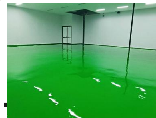
2023 PABRIK SUSU WANAHERANG - EPOXY FLOORING
