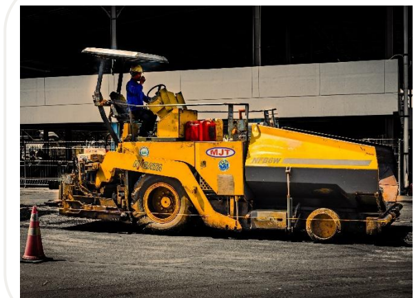
2025 PT. AMERTA INDAH OTSUKA (POCARI SWEAT) – ASPHALT HOTMIX OVERLAY
