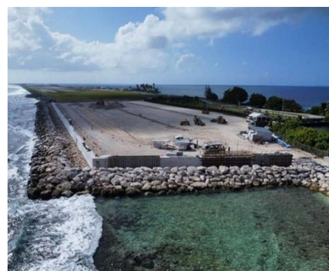
Current progress on JICA reservoir construction
