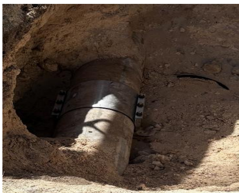
Repair performed on asbestos pipe
