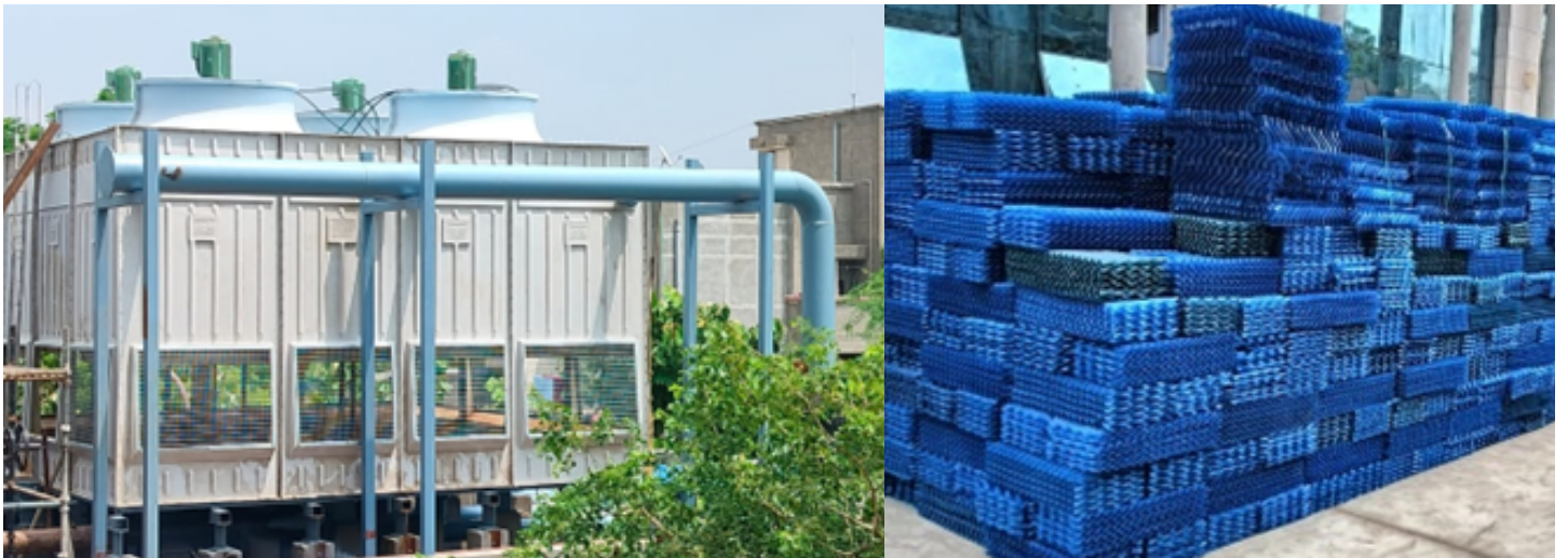
COOLING TOWER INSTALLATION: 2 X 550 TR
